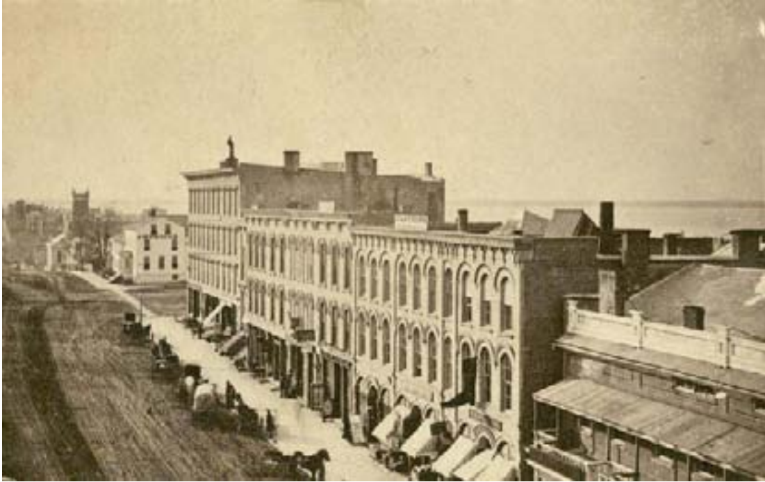
South Pinckney Street 1870, demolished
